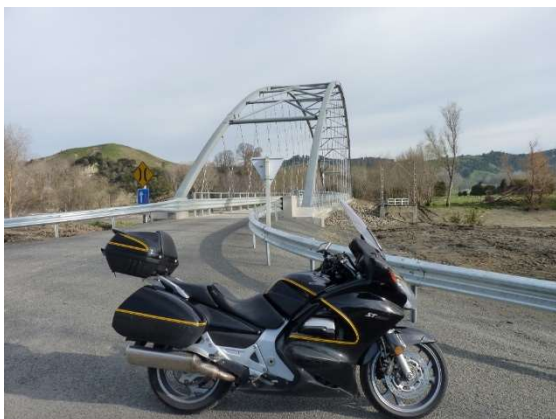
CP13 – Mangamahu Rd Bridge
