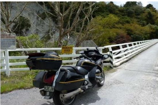
CP3 – Whangaehu River Bridge 202km Waiouru Z*
